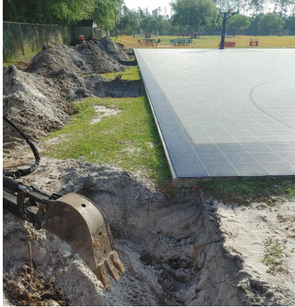
Sports Court roof project underway!
